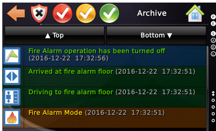
Figure 143: Fire Alarm logbook items.
