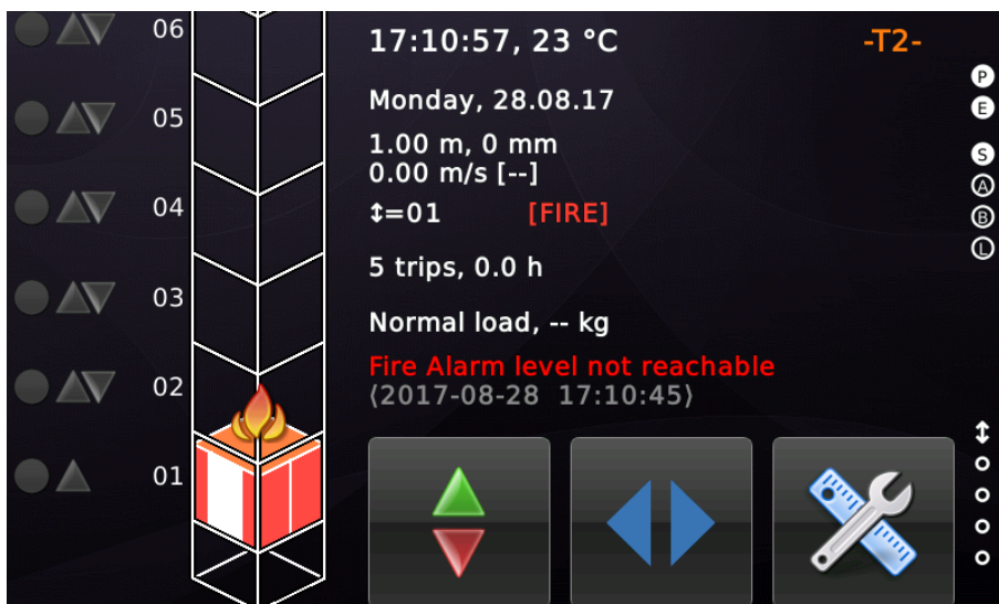
Figure 143: Fire Alarm level not reachable
