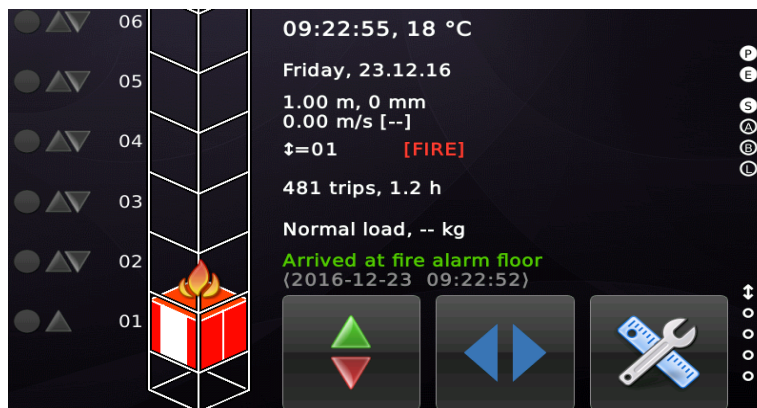
Figure 141: Lift in Fire-Alarm-Operation mode.
